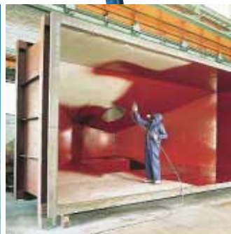
High performance and manageability are demanded in the steel construction industry.
